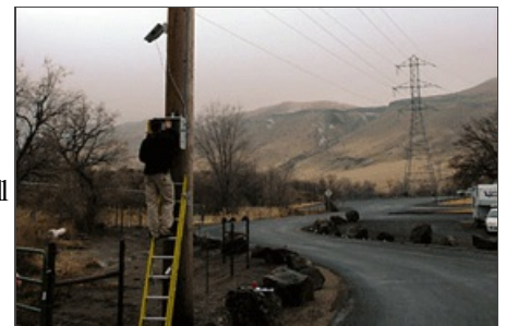
Each weather station measures and records wind speed peaks and averages, wind direction averages, temperature and operating battery voltage.
